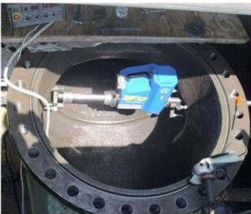
Regeneration of the swing check valve of gas pipelines.
